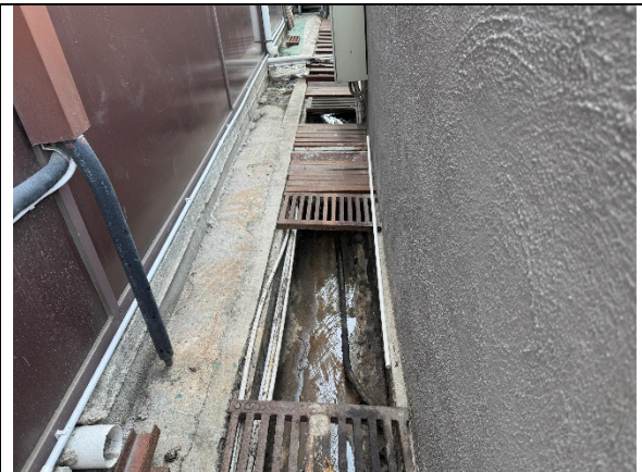
Photo 10 – Existing 525HR surface channel connecting between the existing Catchpit CP7 and the existing terminal manhole of the adjacent site under previously approved Planning Application No. A/YL-TT/596
